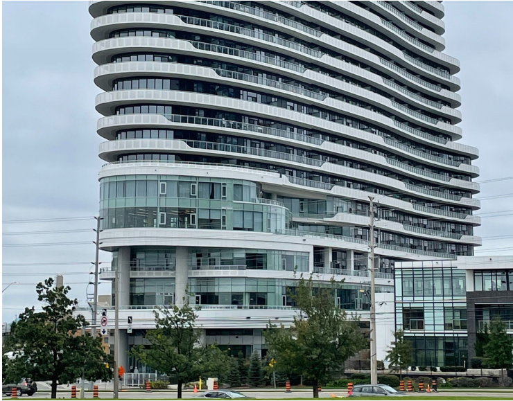
Daniels Erin Mills Arc Condominiums located in Mississauga, Ontario. Photo Credit; The Daniels Corporation
